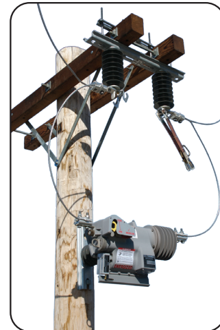
Figure C: Single Bypass Switch Arrangement
